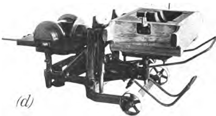
FIG. 255.—Pridmore "Rock-over Drop" Moulding Machine.
